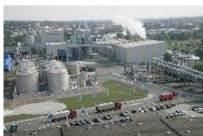
Bioethanol production plant of CropEnergies AG in Zeitz, a subsidiary of Südzucker: The resulting of CO<sub>2</sub> in the production of BioEthanol is microbially bound will be converted to mono- and dicarboxylic acids
